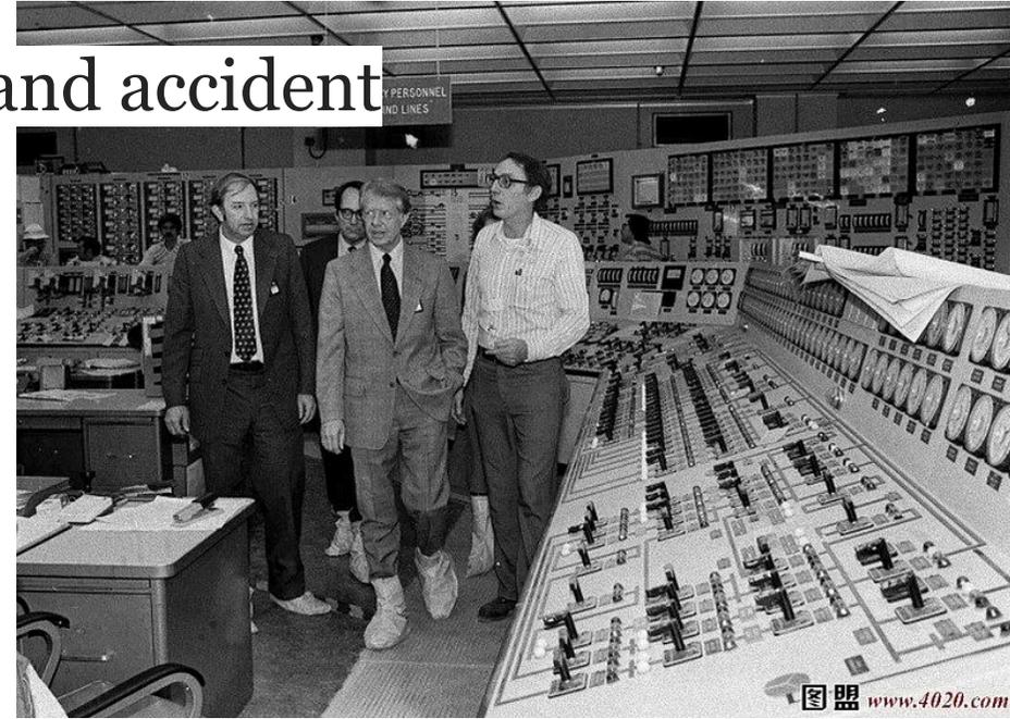
In 1979, the worst nuclear commercial power plant disaster on American soil took place in Pennsylvania. The **status indicator thus gave false evidence of a closed valve**, and when the control room operators were unable to interpret the meaning of the light correctly, they could not correctly diagnose the problem for several hours. By this time, major damage had occurred.
